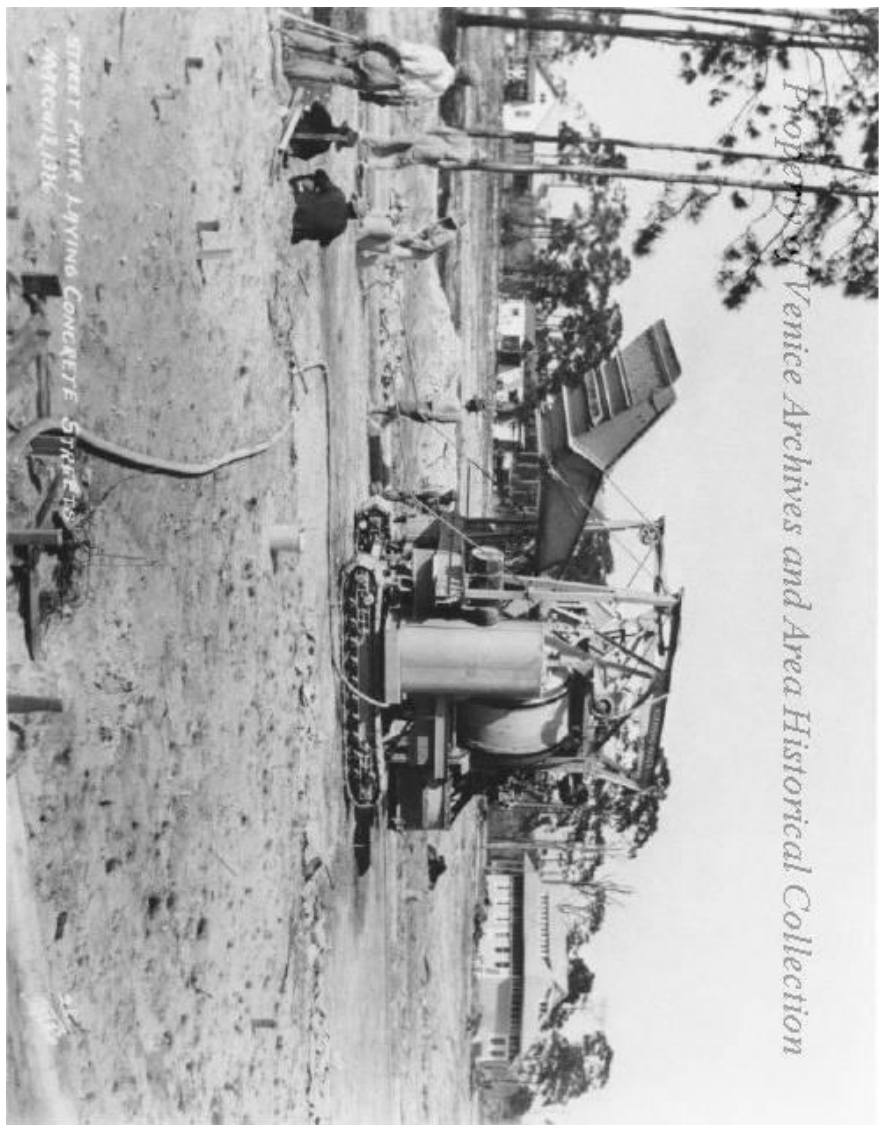
Street paver laying concrete street – March 13, 1926 Photograph by Grover Koons
